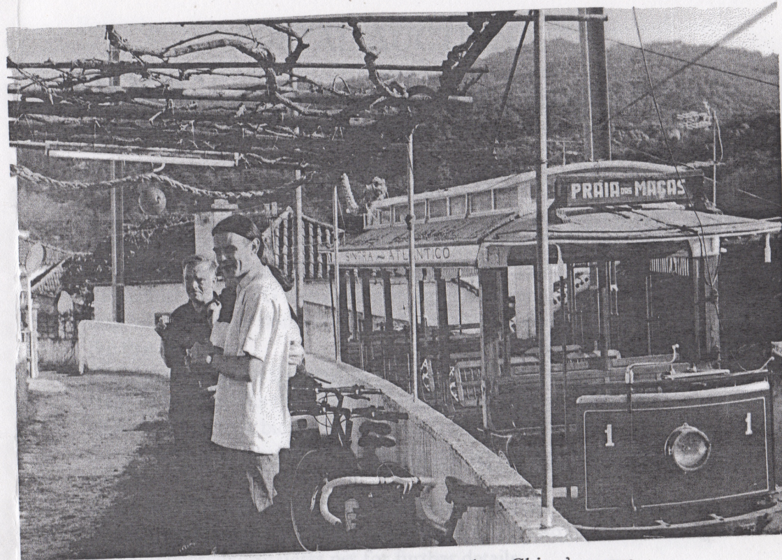
Another check on the state of the track at Chico's curve near Sintra. There was concern that the presence of his wine cellar was deforming the curve at this point. Rectification work seen here in progress. (Visit No. 2).
